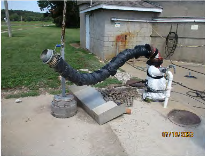
Photo #: 13 Taken by: Joshua Grosvenor Entity: Neosho WWTP Permit: MO0104906 Location: Neosho Shoal Creek Description: Hook up for sludge hauling trucks to load sludge. Date Taken: July 19, 2023 Media: WPCB
