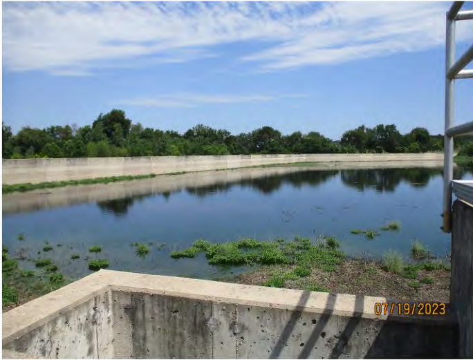
Photo #: 16 Taken by: Joshua Grosvenor Entity: Neosho WWTP Permit: MO0104906 Location: Peak flow basin Description: Peak flow basin, eight million gallons. Date Taken: July 19, 2023 Media: WPCB
