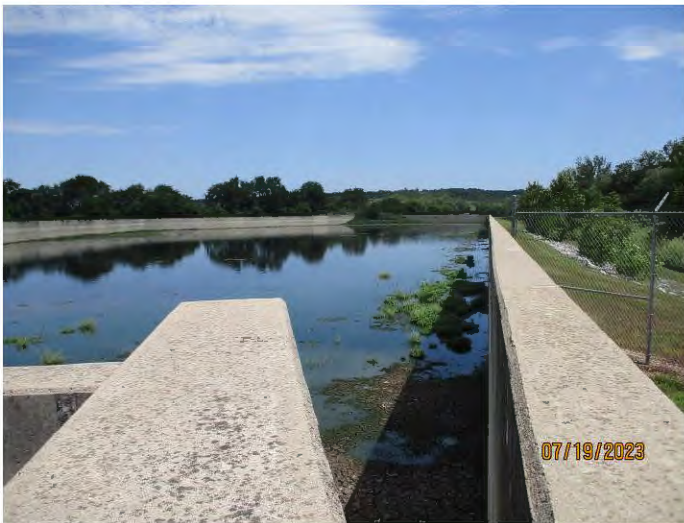
Photo #: 17 Taken by: Joshua Grosvenor Entity: Neosho WWTP Permit: MO0104906 Location: Peak flow basin Description: Peak flow basin, eight million gallons. Date Taken: July 19, 2023 Media: WPCB
