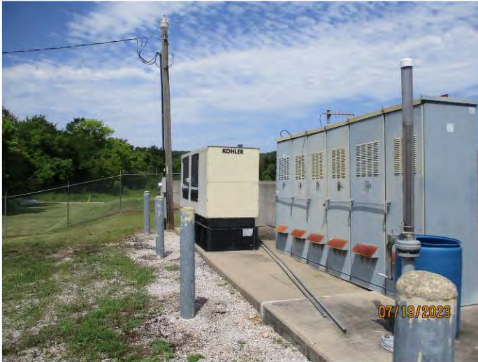
Photo #: 19 Taken by: Joshua Grosvenor Entity: Neosho WWTP Permit: MO0104906 Location: Peak flow basin Description: Peak flow basin backup generators, exercised regularly. Date Taken: July 19, 2023 Media: WPCB
