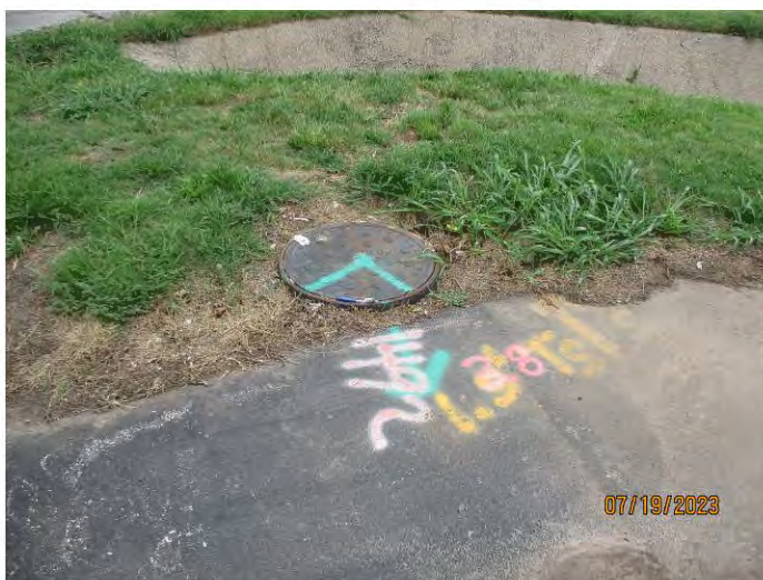
Photo #: 27 Taken by: Joshua Grosvenor Entity: Neosho WWTP Permit: MO0104906 Location: S Neosho Boulevard and W South Street Description: Manhole with the greatest frequency of overflows, during high flow events. Date Taken: July 19, 2023 Media: WPCB
