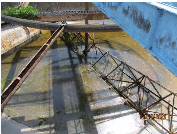
Photo #: 9 Taken by: Joshua Grosvenor Entity: Neosho WWTP Permit: MO0104906 Location: Neosho Shoal Creek Description: Clarifier, currently under repairs. Date Taken: July 19, 2023 Media: WPCB
