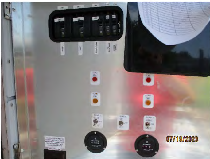
Photo #: 21 Taken by: Joshua Grosvenor Entity: Neosho WWTP Permit: MO0104906 Location: Jay Drive Lift Station Description: Lift station control panel with inspection log visible. Date Taken: July 19, 2023 Media: WPCB
