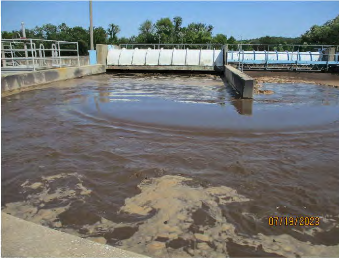
Photo #: 4 Taken by: Joshua Grosvenor Entity: Neosho WWTP Permit: MO0104906 Location: Neosho Shoal Creek Description: Oxidation Ditch Date Taken: July 19, 2023 Media: WPCB
