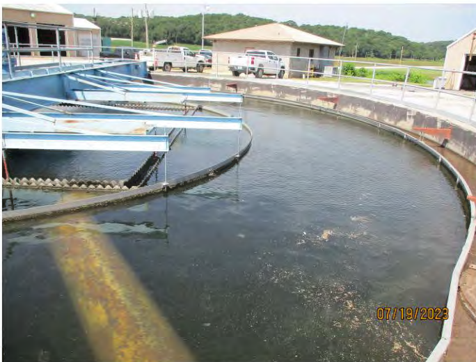
Photo #: 6 Taken by: Joshua Grosvenor Entity: Neosho WWTP Permit: MO0104906 Location: Neosho Shoal Creek Description: Operational clarifier. Date Taken: July 19, 2023 Media: WPCB
