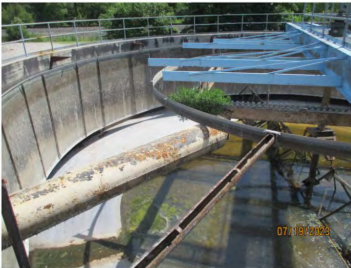
Photo #: 8 Taken by: Joshua Grosvenor Entity: Neosho WWTP Permit: MO0104906 Location: Neosho Shoal Creek Description: Clarifier, currently under repairs. Date Taken: July 19, 2023 Media: WPCB
