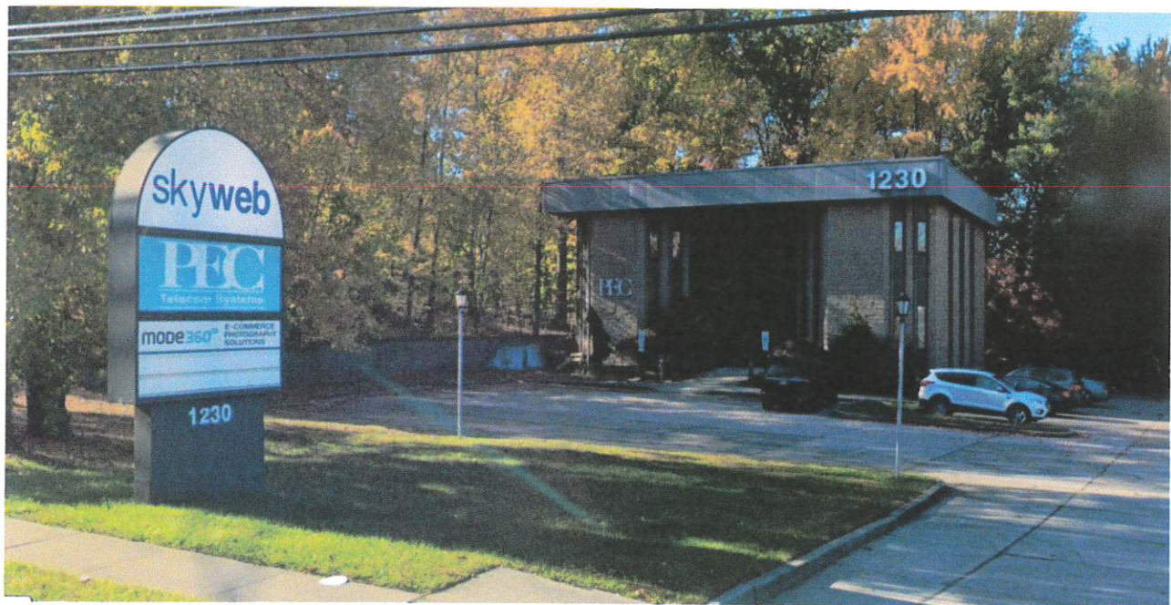
Figure 1. PEC Building located in Aberdeen, New Jersey
