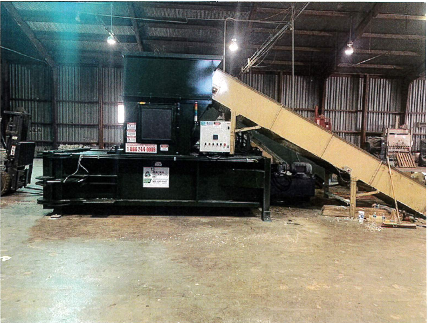
CITY OF PLAINVIEW TEXAS 2021 THB-6048 INSTALLATION
